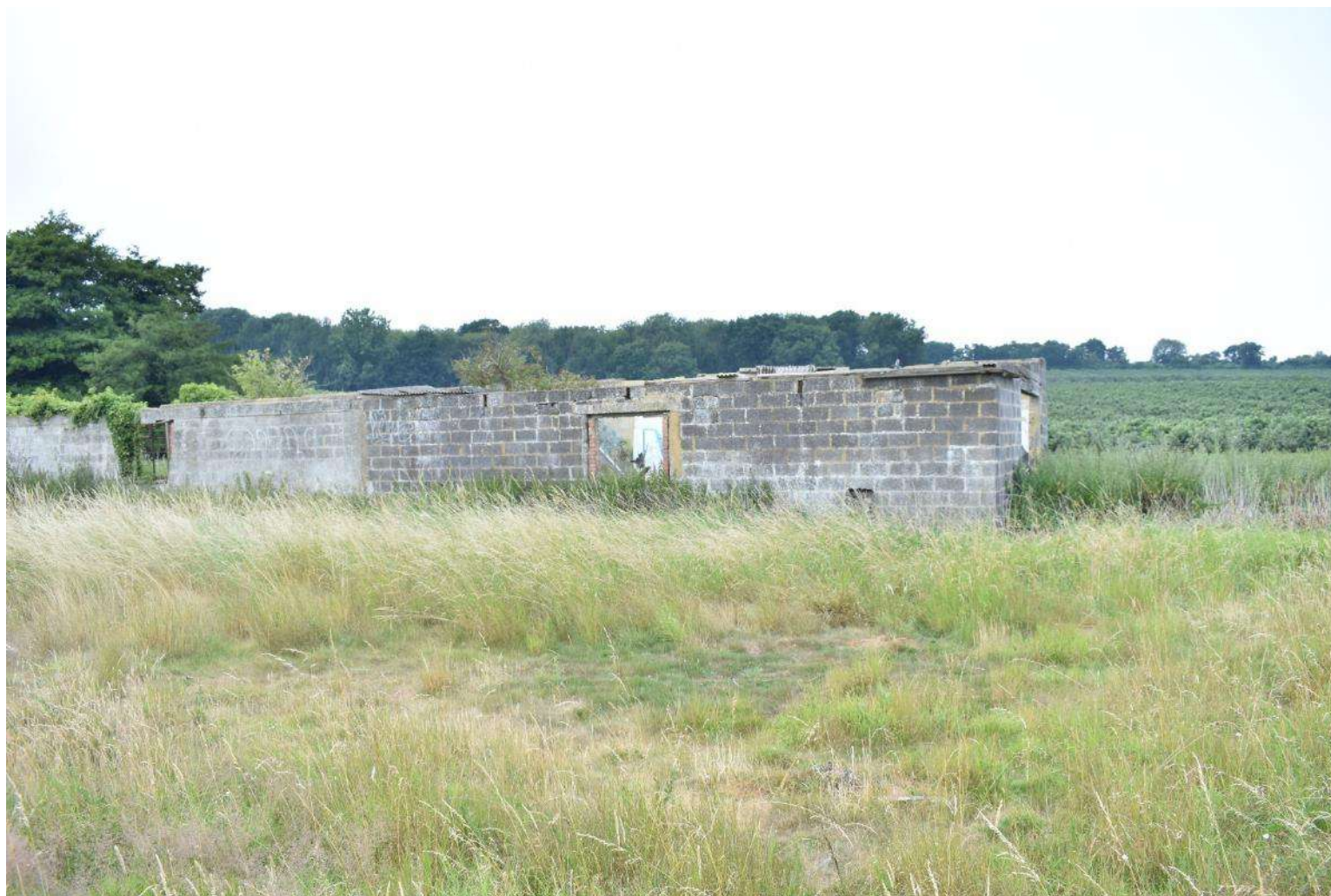
Plate 8: View of the building to be demolished (looking west, north west)
